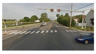
In addition, as part of the new sidewalk project, DelDOT installed a High-Intensity Activated Crosswalk (HAWK) signal at the intersection of SR 8, Heatherfield Way, and the east entrance to the high school as shown below in Figure 13. The HAWK signal is a traffic signal that turns to red upon activation by a pedestrian. The signal stays dark unless activated. The HAWK signal pro-vides a safe signalized crossing for pedestrians crossing SR 8 to the high school.
